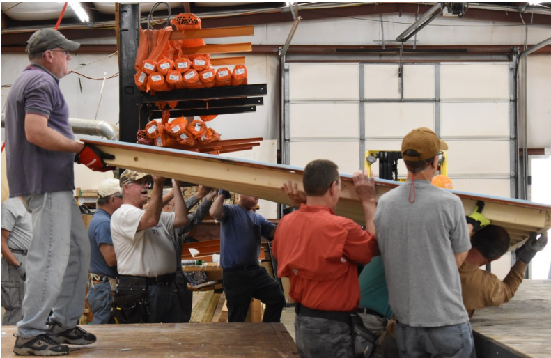
Volunteers load a newly-built wall on the trailer.
