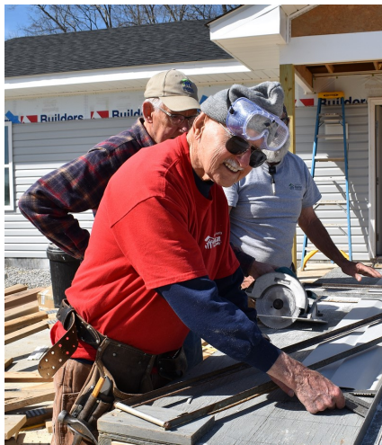
Bill Durant works on siding a house.
